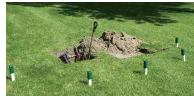
Mark off repair areas
